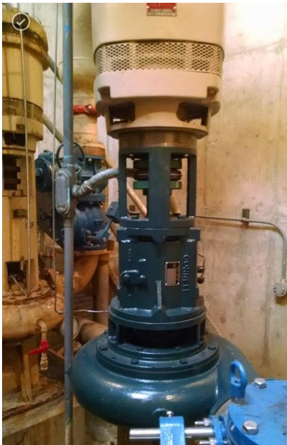
Influent Pump No. 4 w/ adapter plate and motor attached.
