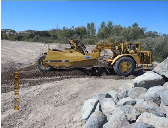
Final Grading Activity
