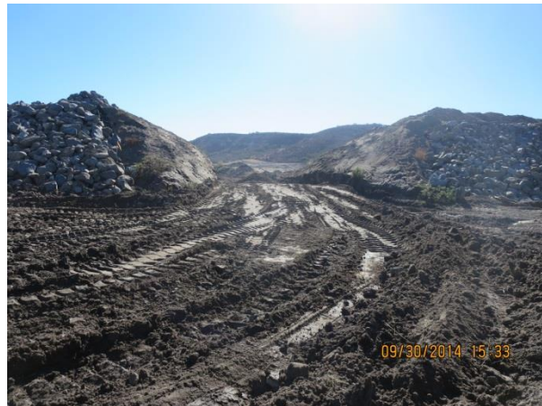
Diversion channel before final grading
