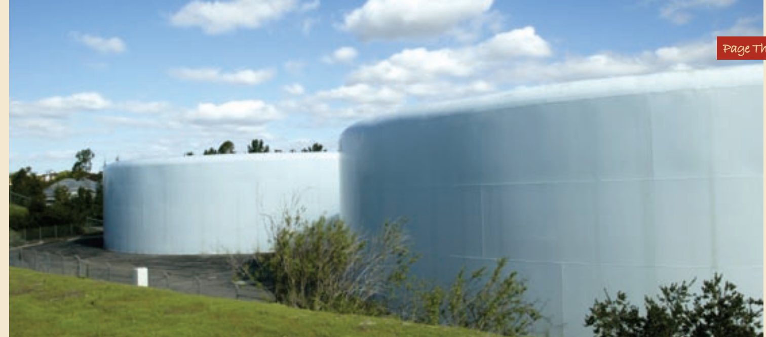
The Trabuco Ridge Reservoirs serve homes within Rancho Santa Margarita.
