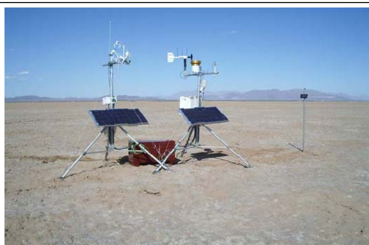
Figure 1. EC Instrumentation and Meteorological Towers Installed on Bristol Dry Lake
